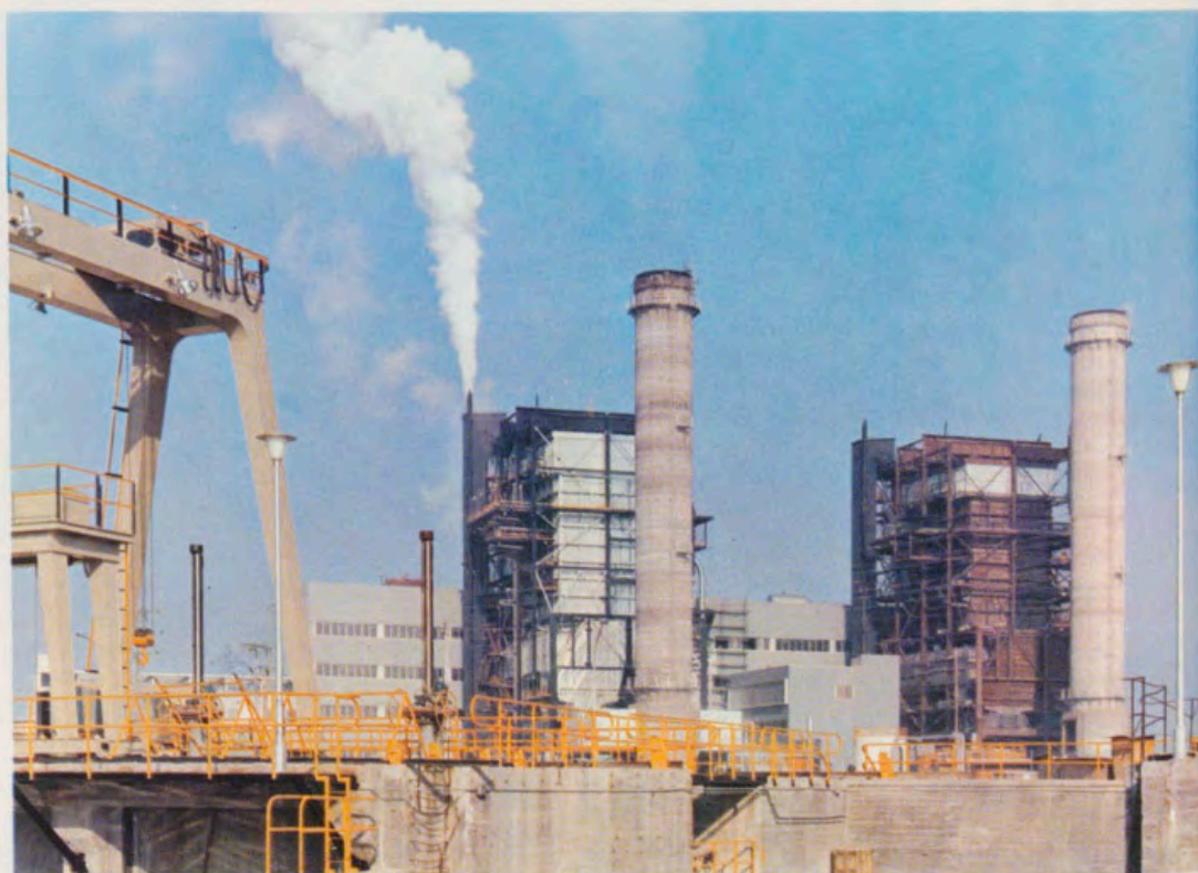
CENTRAL TERMICA DE ACECA
